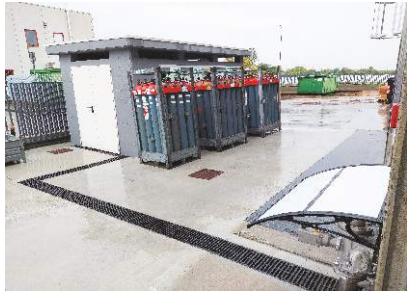
ATEX compliant hydrogen supply and reduction line for packaged cylinders at 200 BAR
