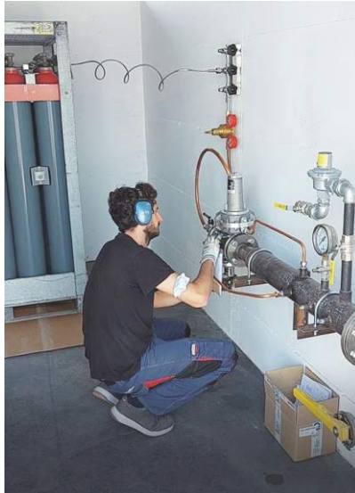
ATEX compliant hydrogen supply and reduction line for packaged cylinders at 200 BAR
